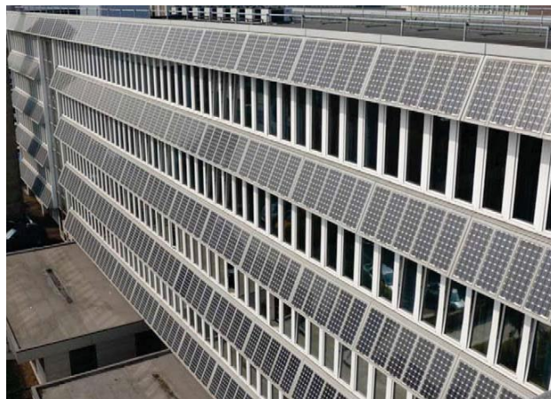
Figure 2.1 The 40 kWp facade of the Northumberland building at Northumbria University, United Kingdom, which uses the crystalline silicon solar modules manufactured by BP Solar (Saturn modules) (Miles, Zoppi, & Forbes, 2007).
