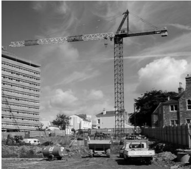
Figure 1.1 Rotary tower crane in a construction.
