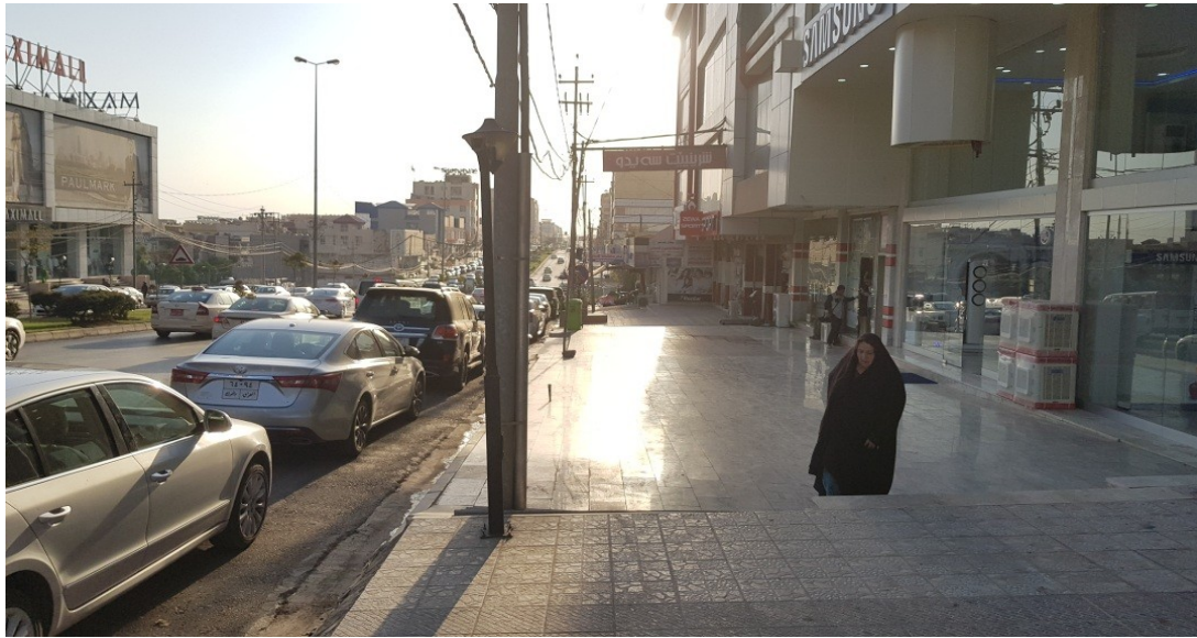
Figure 1.1: KRO Street Walkway Without or Inadequate Streetscape Elements Source: Field Observation, 2017
