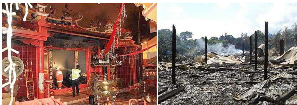
Figure 1.1: Aftermath of fire in Ho Ann Kiong Temple (left) and Punan Bah Longhouse (right) (Source: thestar.com.my)
