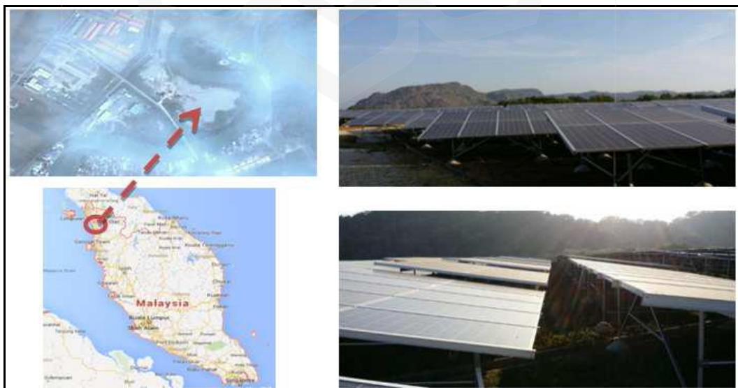
Figure 1 Solar power plant (solar farm) in Perlis, Malaysia (Kassim et al., 2015).
